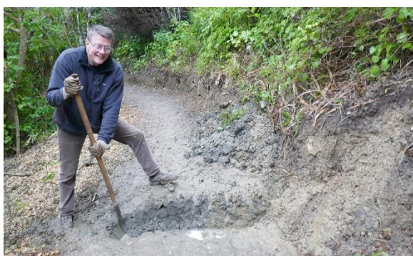
Track man Dick: another day, another culvert!
